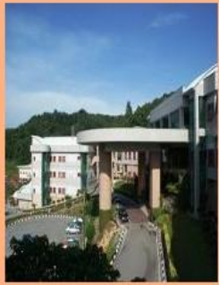
Side view of the AELB Headquarters, Selangor
